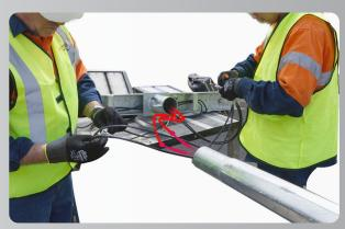
a. Feed the cables through the hole in the bottom of the crossarm.
