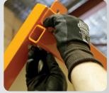
Bolt panels to the support arms, checking the tension of each bolt to ensure it is secure.
