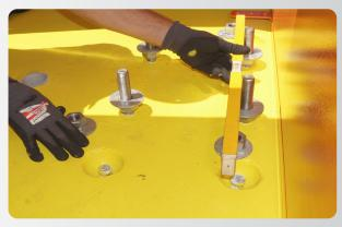
Remove top nut and washer from mounting bolts. Set height of each nut, so there is a minimum 42mm clearance between block and the top of the washer. The nuts then need to be levelled to ensure the pole will mount flat. This can be checked with a spirit level on the top of the washers.
