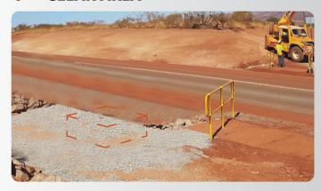
Clear an area that is suitable and level for the safe installation of the Earthtrack Solar Light Tower.
